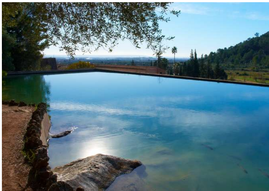
The Raixa cistern or washhouse is one of the largest in the Serra de Tramuntana.
