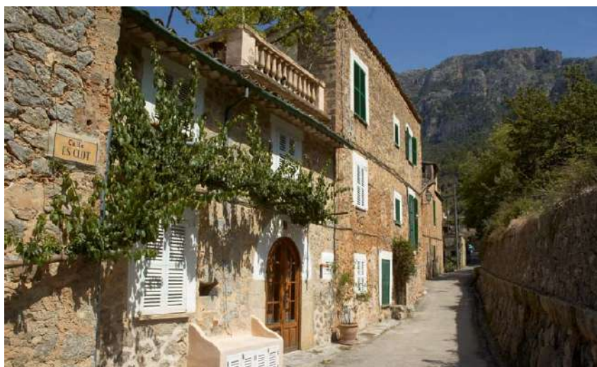
View of a street in the village of Deià. Stone is omnipresent in the urban landscapes of the Serra de Tramuntana.
